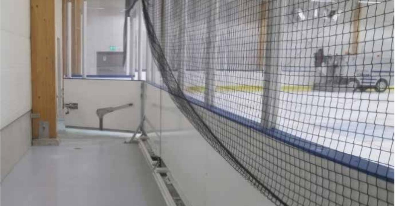
**Figure 21.** Dasher boards fulfil important functions, not the least in terms of safety.
