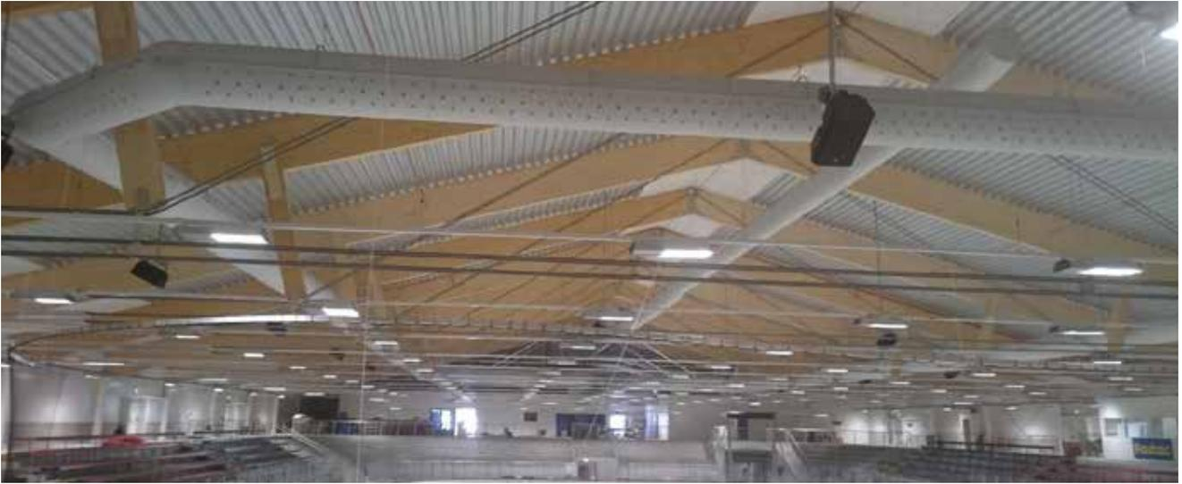
**Figure 47.** Textile ducts in an ice rink where dry air is distributed over the ice and “comfort air” to the stands.
