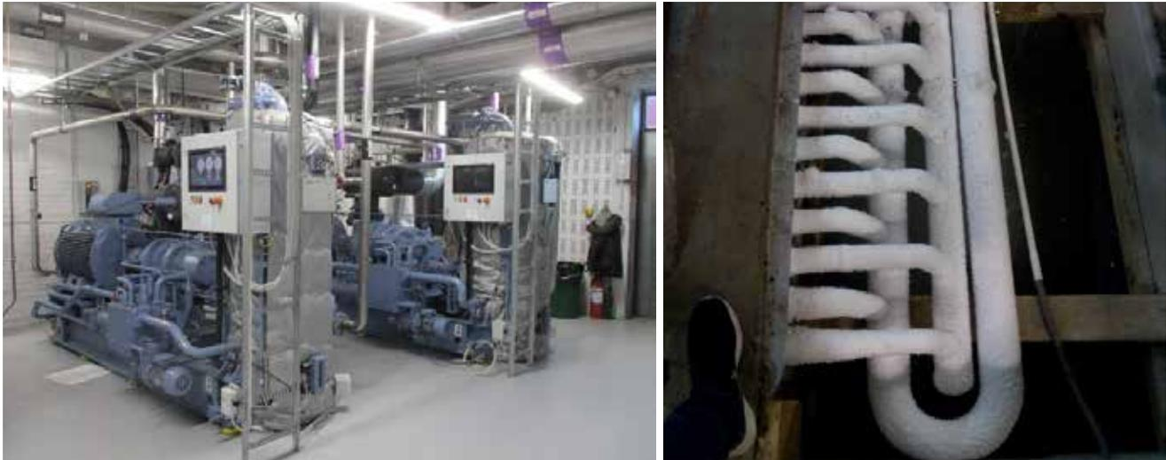
**Figure 22.** The primary system (on the left) involves a primary refrigerant, it cools a fluid in a secondary system (on the right) that circulates in the rink pipes.
