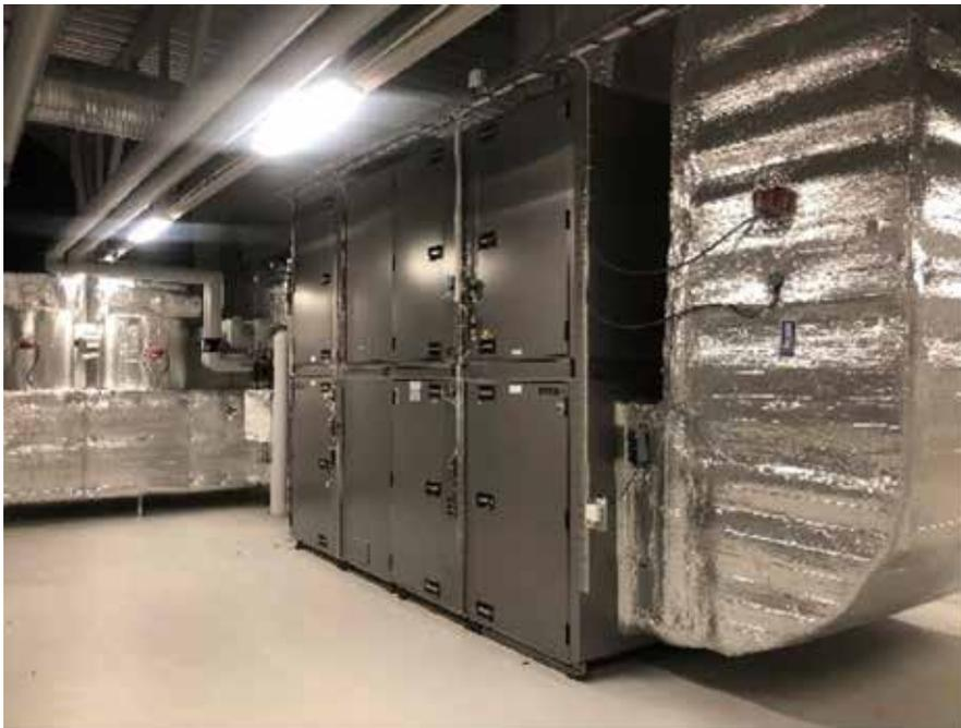
**Figure 49.** Example of a central air handling unit in an ice arena, the unit is located in a technical room.
