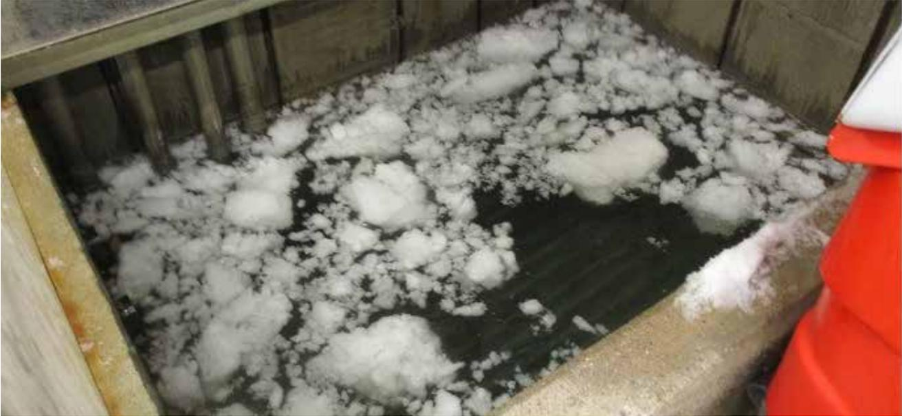
**Figure 57.** By recycling the resurfacing water from the melting pit, the water management of an ice arena can be significantly improved.
