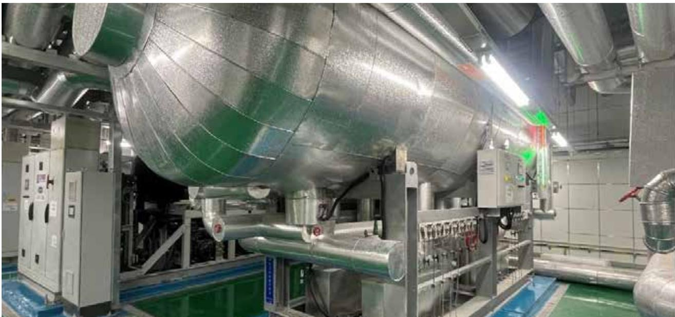
**Figure 33.** CO<sub>2</sub> receiver in a large ice arena where CO<sub>2</sub> is circulated in the rink piping.
