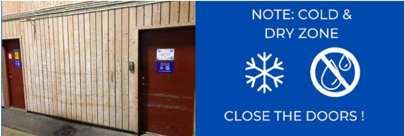
**Figure 16.** Doors between the cold space and heated spaces must be with high thermal resistance, hermetically sealed and normally kept close.
