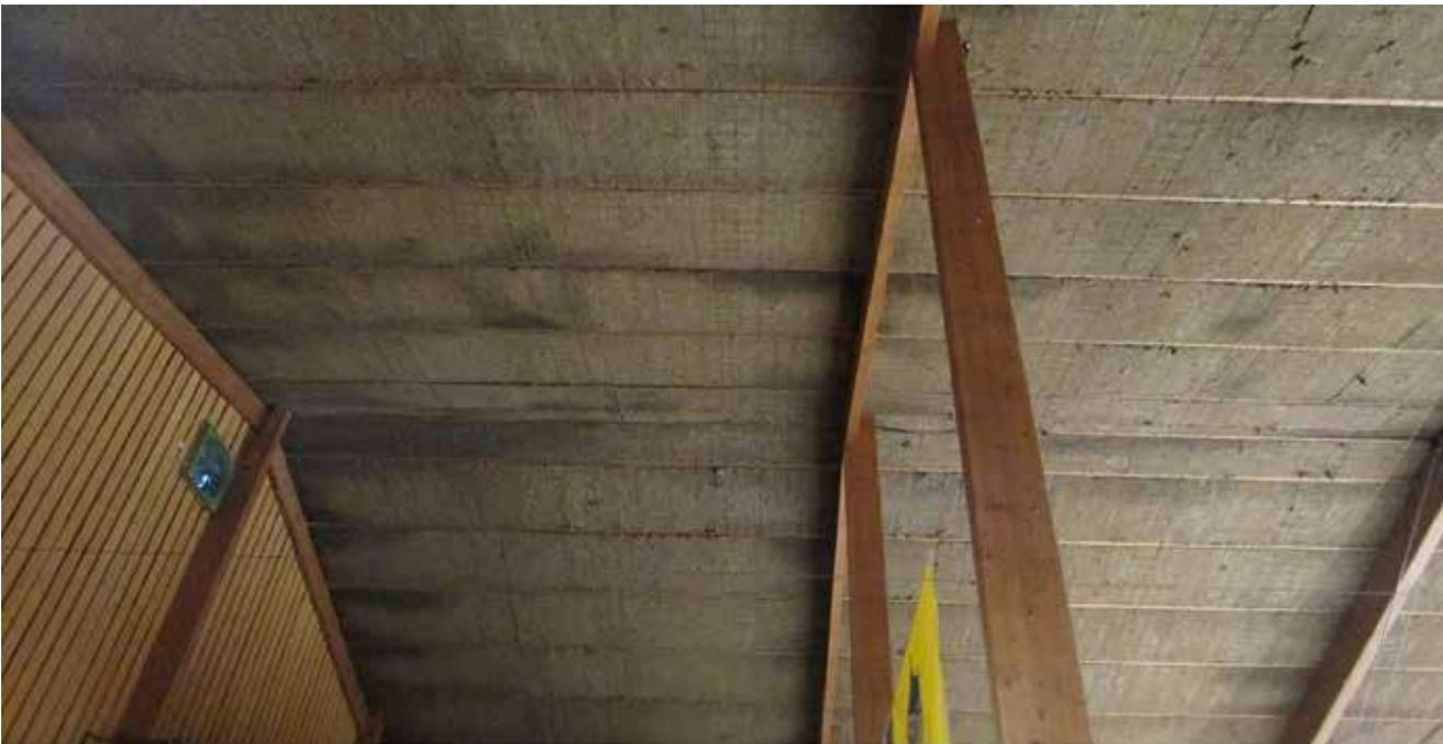
**Figure 13.** Air leakage traces near the joint between roof and wall.
