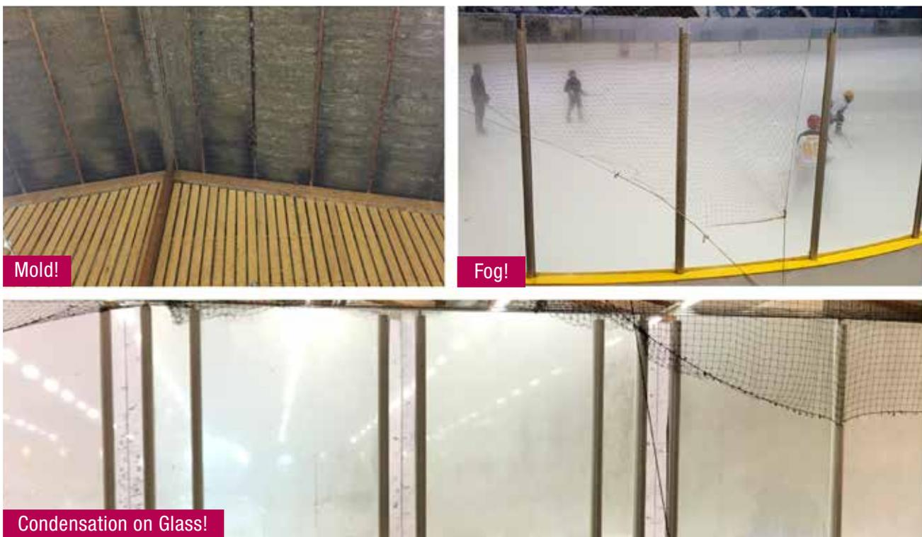
**Figure 39.** Moisture problems are known in many ice rinks. Solution to keep the indoor humidity at acceptable level must be used.
