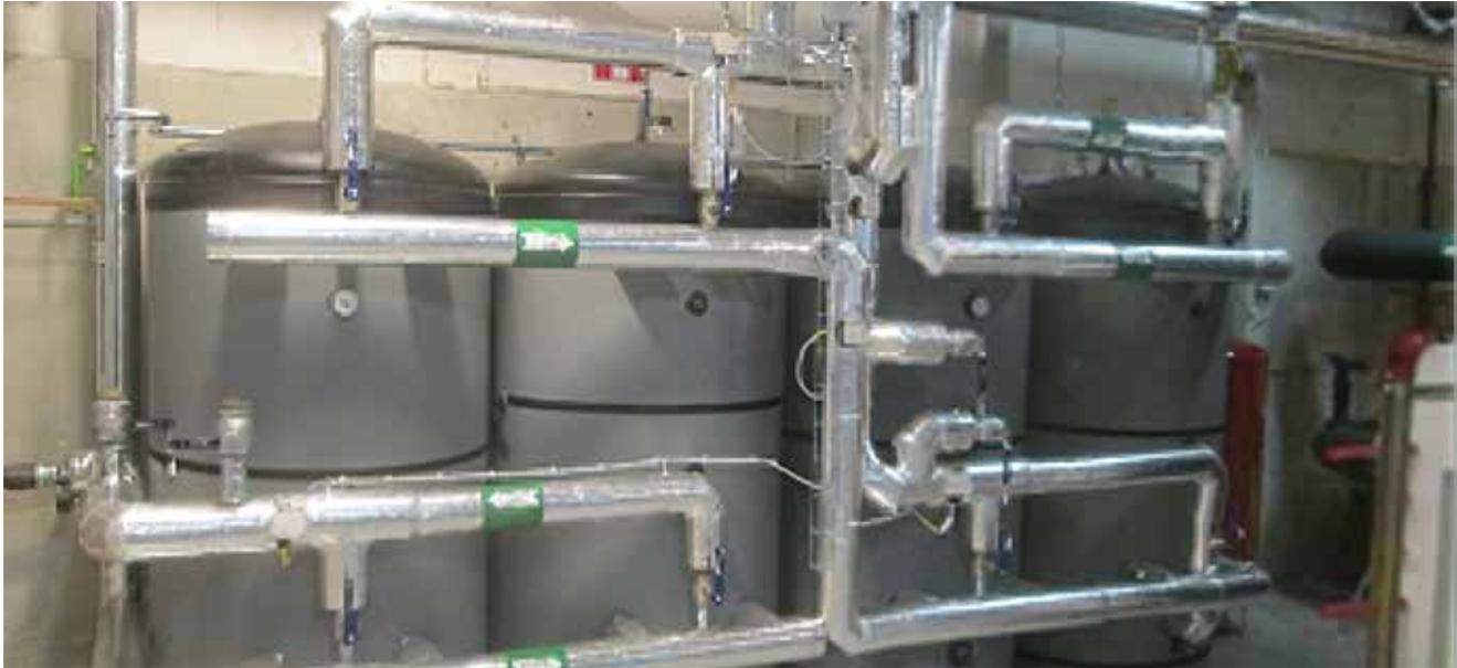
**Figure 37.** Groups of accumulator tanks with coils for tap water pre- and post- heating.
