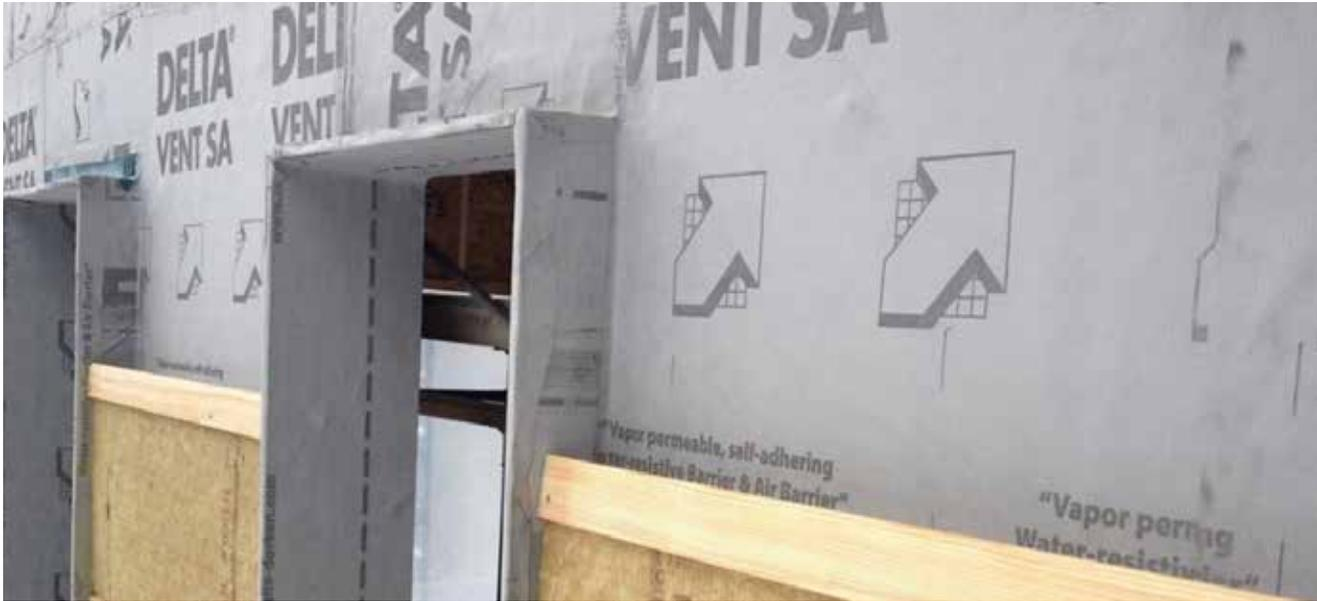
**Figure 14.** Polyethylene self adhering air barrier (Delta Vent, 2019)
