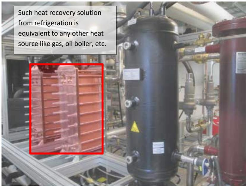
**Figure 36.** Heat recovery from modern refrigeration makes such systems a 2-in-1 solutions as they provide both cooling and heating.
