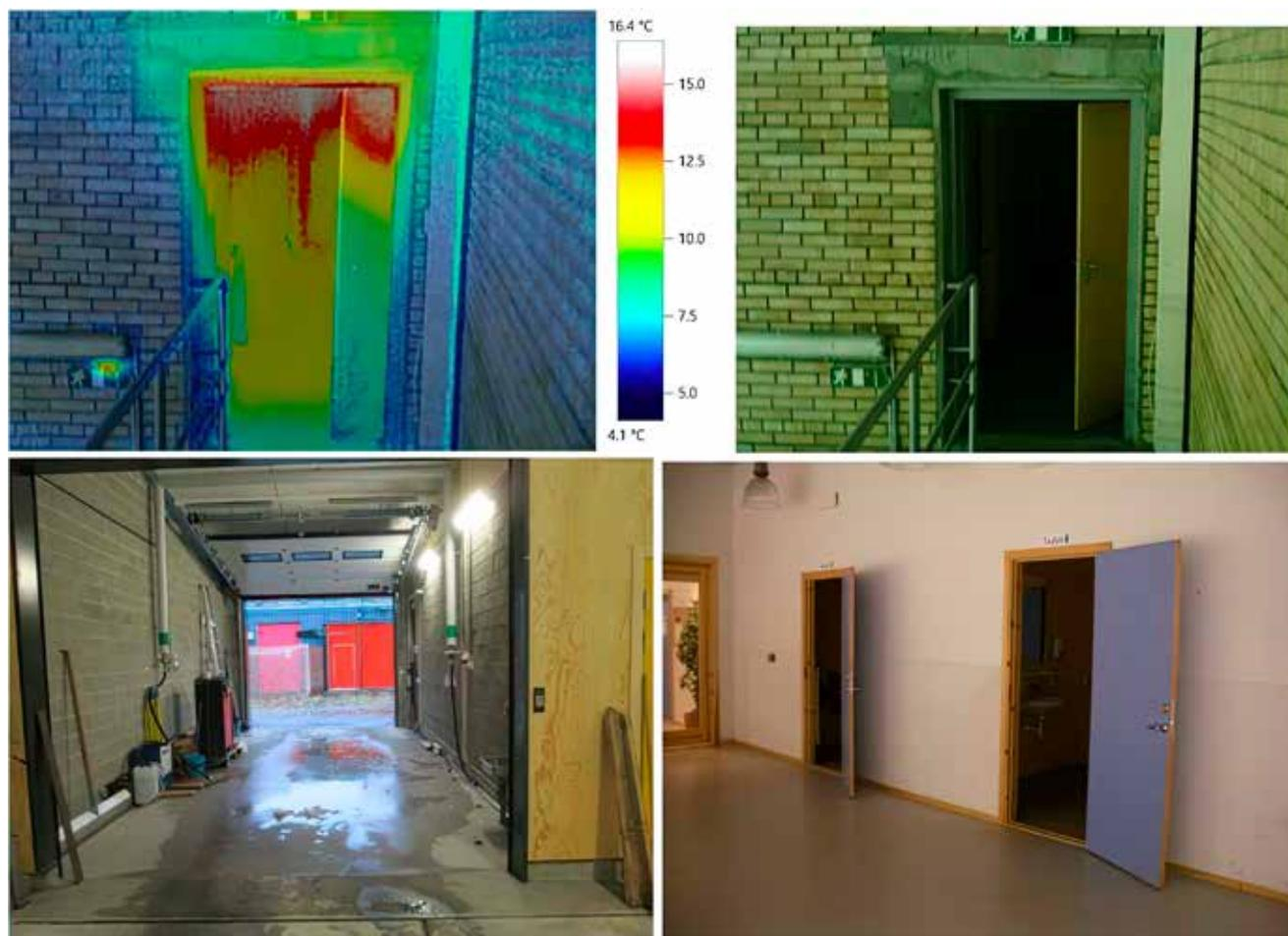
**Figure 15.** Open doors either directly towards outdoors, or between comfort and arena zone cause significant energy and moisture influx into the arena room. In addition, basic uninsulated wooden doors are found between climate zones in some ice rinks which is not an optimal solution.
